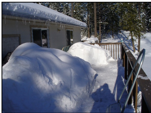
From the roof to the deck!
