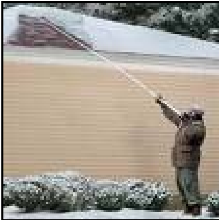
Roof Snow rake in action
